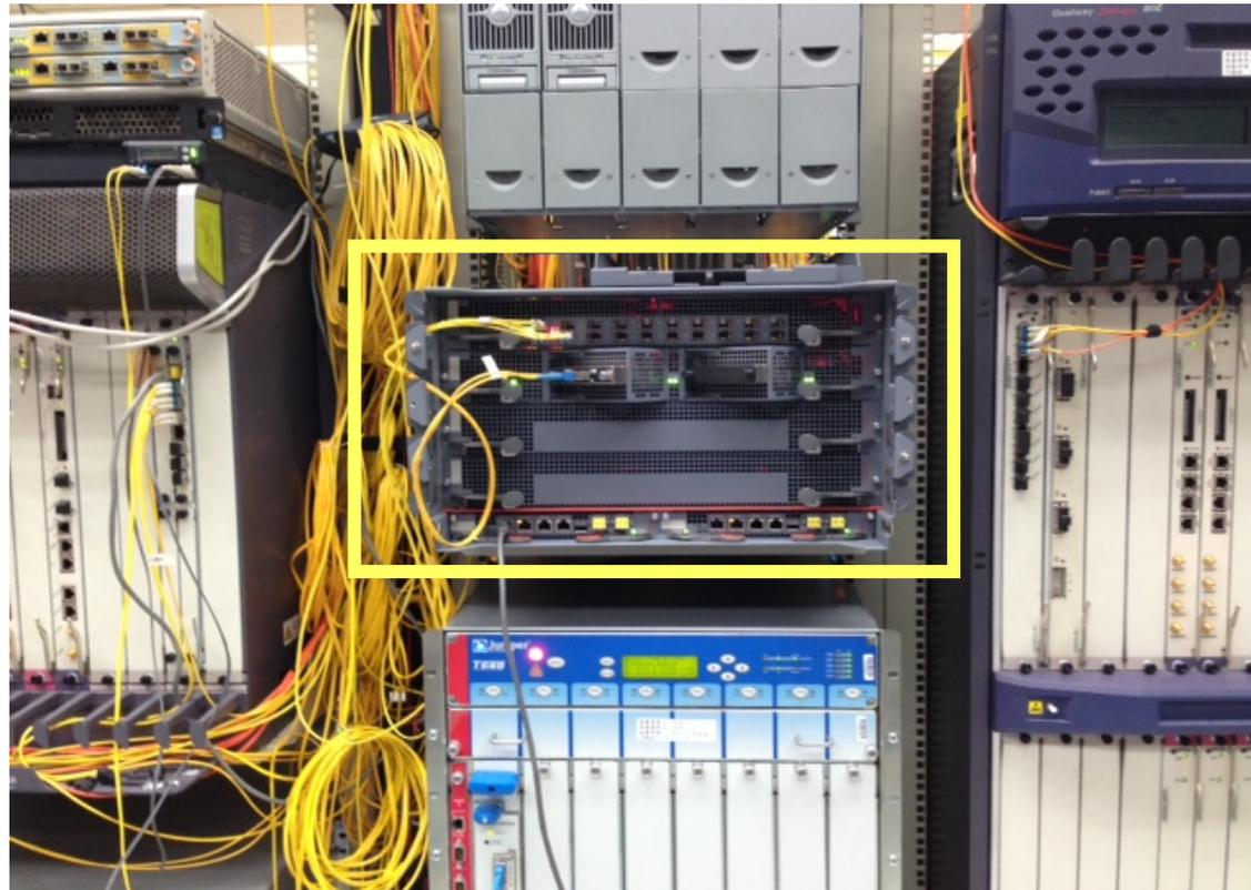
Compass EOS (The chip-to-chip direct silicon-to-photonics solution ) for testing
